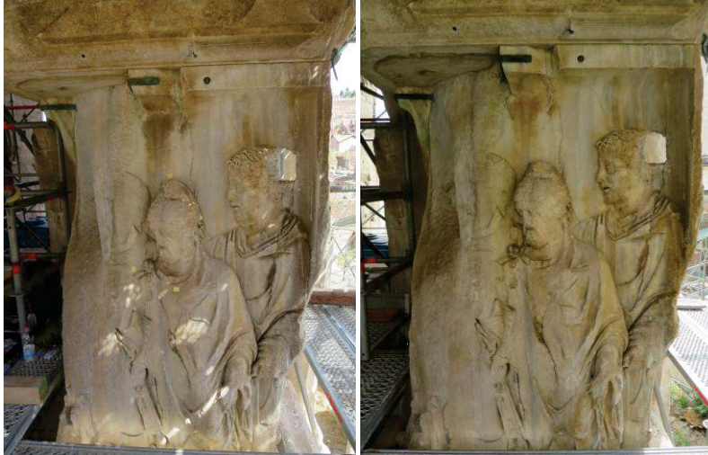
Fig. 1: West plane of the plinth before (left) and after (right) the biom mineralisation treatment.
